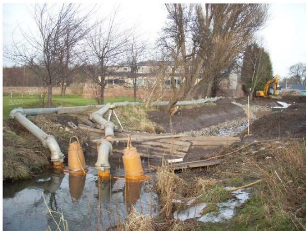
Plate 8: Full isolation – over pumping/siphon
