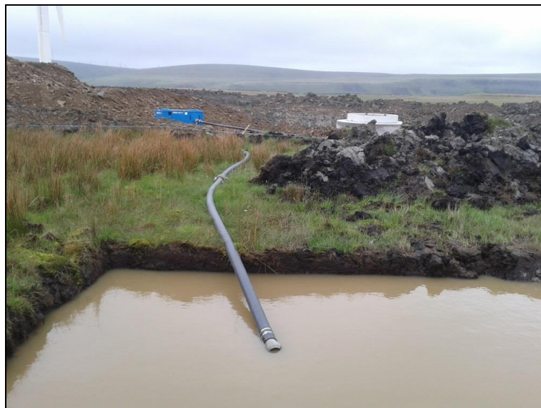
Plate 6: Typical 'Siltbuster' and settlement lagoon
